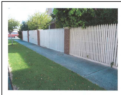
Brick Piers with timber inserts
