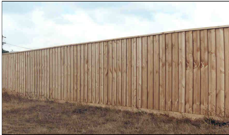
Figure 2: Standard Boundary Fencing
