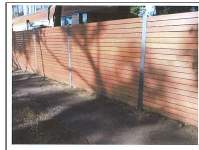
Exposed steel posts with merbau inserts
