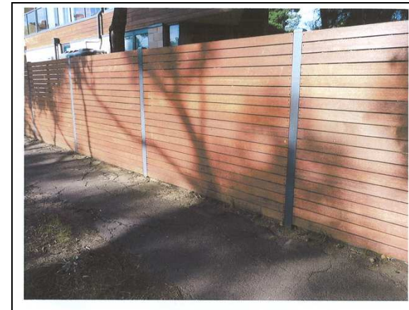
Figure 6: Fencing Adjoining Pedestrian Link
