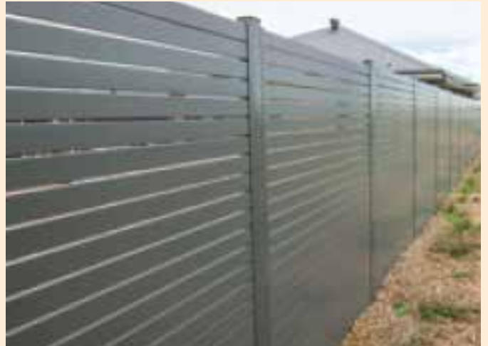
Corner lot fencing
